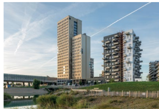
The 84-metre-high wooden high-rise, known as “ Hoho ” (at left in the picture), in Seestadt Aspern near Vienna (Austria), consists of three wooden high-rises arranged in an L-shape. The tallest of the three stands at 57 metres and is positioned at the angle between the two shorter buildings, which are 40 metres in height.
