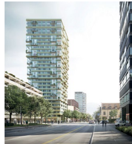
With the residential high-rise „ Project Pi ” in Zug will be the tallest timber high-rise in Switzerland to date, rising 80 metres into the sky by 2024. The high-rise is divided into four segments, each slightly receding from top to bottom, giving the building a subtle tapering effect towards the base.
