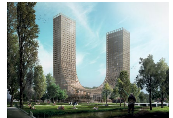
The sculptural U-shape of “ The Dutch Mountains ” is formed by two towers that are seamlessly connected at the base – one 130 m high, the other 100 m high. The elegant lines of the façade extend into a roof structure made of laminated wooden beams, which will be visible from the central interior.
