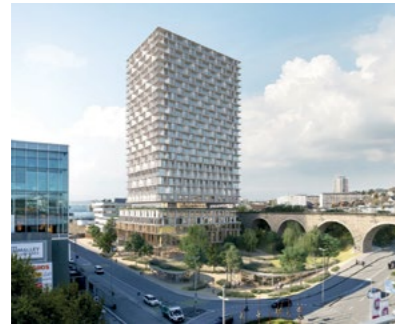
On the outskirts of Lausanne (Switzerland), the 85 m high Tilia Tower is in the planning. The wood (hybrid) high-rise is part of an urban development project.
