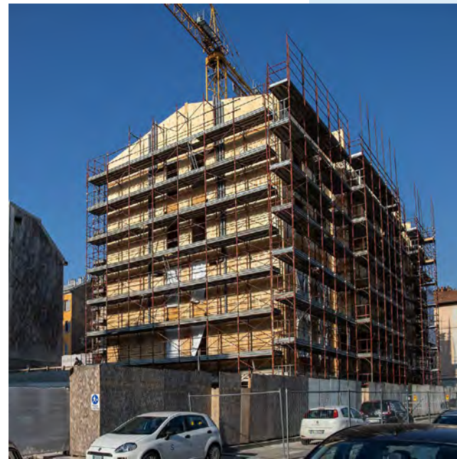
In the heart of Milan, a multi-storey residential complex is being built as a solid timber construction, exclusively using Pfeifer CLT.
