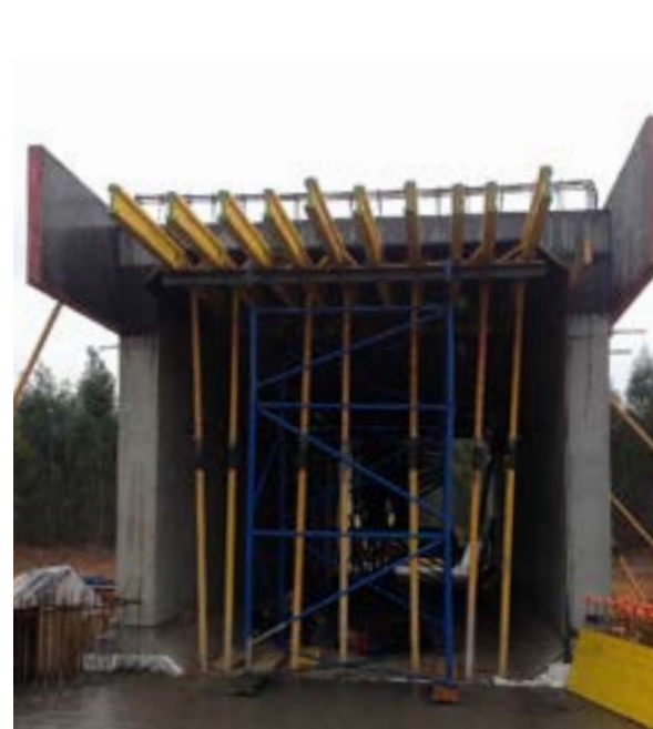
In use: formwork beams by Pfeifer in the construction of the first high-speed train in Africa.
